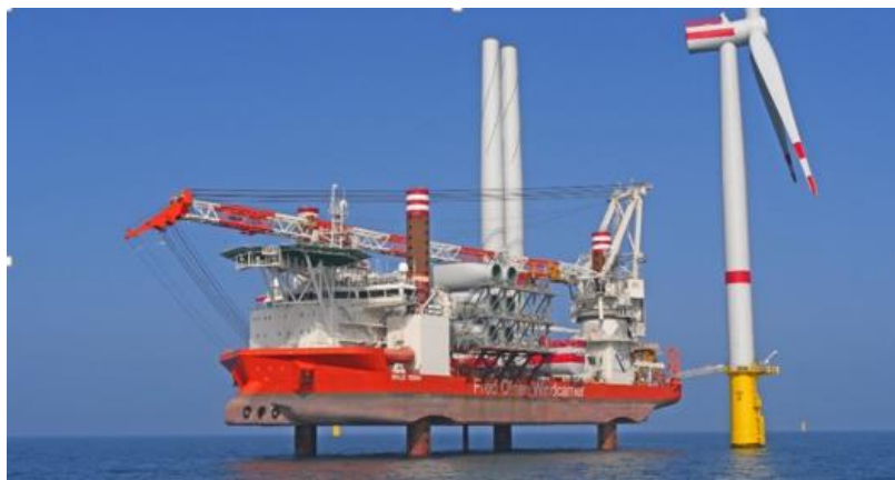
Three modern transport and installation vessels (T&I) and seven crew transfer vessels
