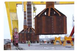
Providing the innovative Mono Bucket Foundation for offshore wind turbines
