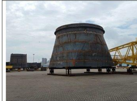
Pedestal adapter machining completed, secondary steel outfitting to start
