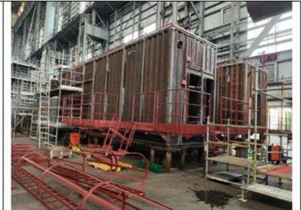
E-room welding being completed
