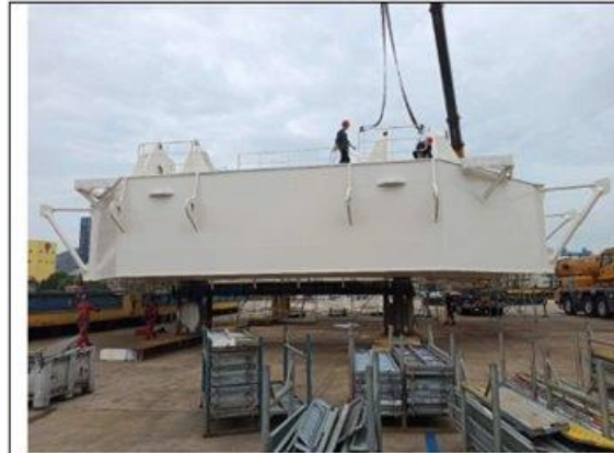
Slew platform painting completed and outfitting started
